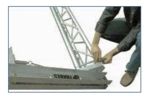
Now assemble the vertical trusses and lock the head on.
